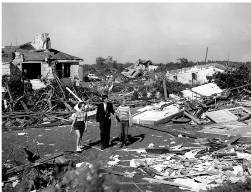
Sen. John F. Kennedy, Massachusetts, center, with two companions, inspects tornado damage in Shrewsbury, Mass., June 10, 1953. The F4 tornado caused 94 deaths, 1,300 injuries, and destroyed or damaged 4,000 buildings and hundreds of cars in Central Massachusetts, which begins the New England tornado alley.
